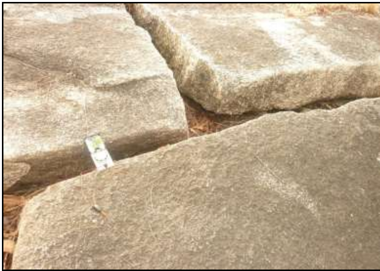
Figure 25: Open exfoliation fractures in porphyritic granite (06°55'58"N, 09°15'49"E).
